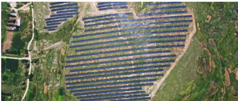
Aerial View of the 7.767 Mw Power Station Project in Jiaoyu Town, Tai'an, Shandong
