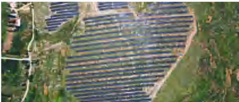
Aerial View of the 7.767 Mwp Power Station Project in Jiayu Town, Tai'an, Shandong
