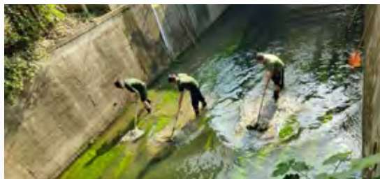
Risen Energy Carries Out Cleaning and Maintenance Work on the Adjacent River
