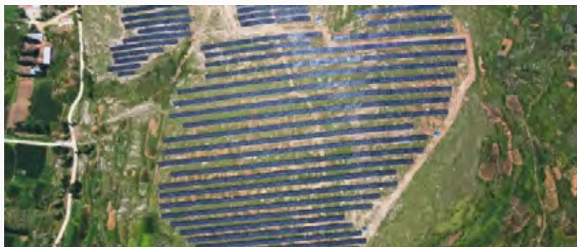
Aerial View of the 7.767 Mwp Power Station Project in Jiayou Town, Tai'an, Shandong
